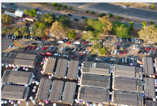
Exhibit 10. Shops in Wuse Market adopted on-site solar
